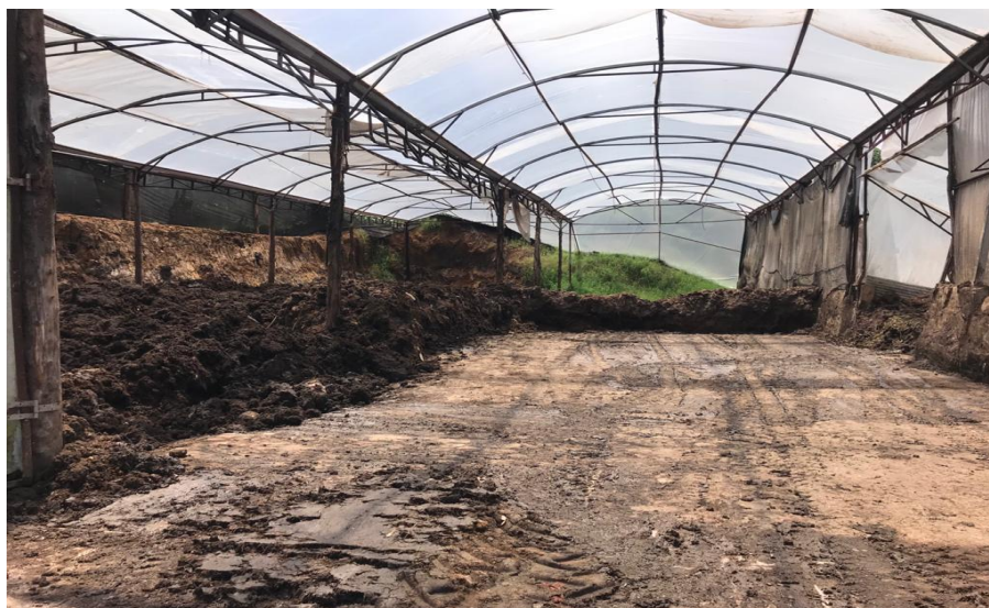
Temporary storage area for maturing product.
